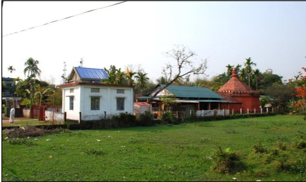
Figure 1. View of the monument from south-east
